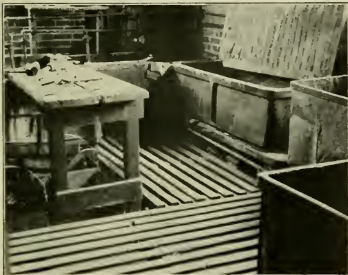
Lacquer Room with Tanks for Cleaning.
